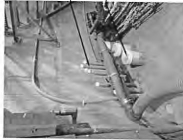
4 EXISTING CONDUIT ENTRY INSIDE OF WATER TANK
