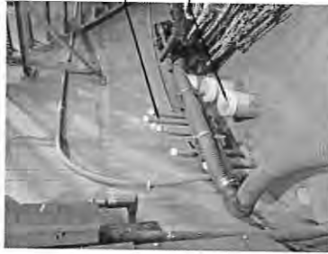
4 EXISTING CONDUIT ENTRY INSIDE OF WATER TANK
