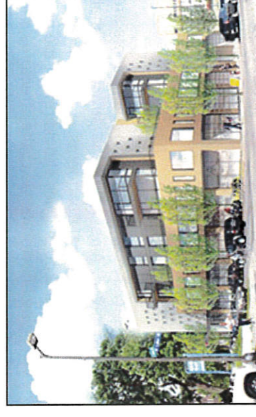
Building Mass is reduced by breaking the building up into smaller sections and “stepping-back” levels above the ground floor. Source: www.minnpost.com
