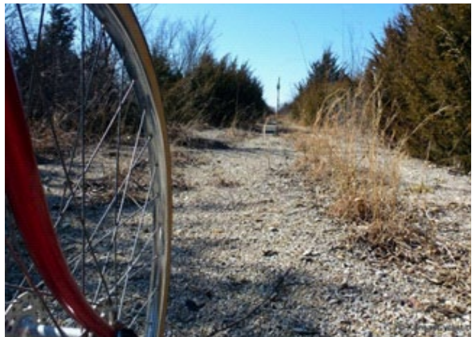
Uncontrolled weed growth through trail surface.
