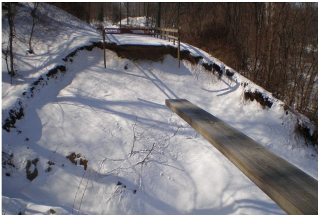
Culvert failure, Manhan Rail Trails, MA.
