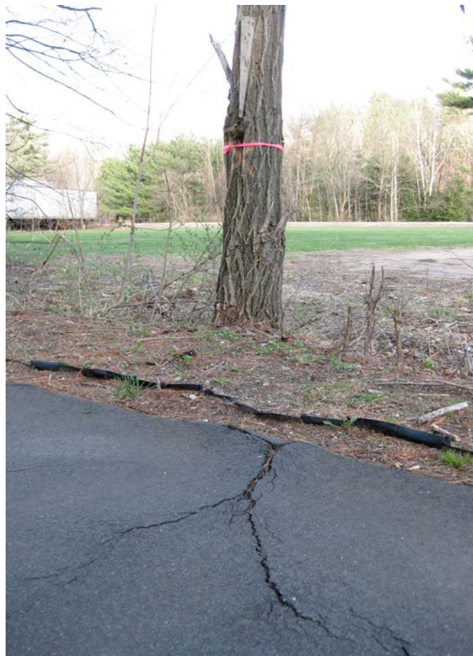
Tree root damage Manhan Rail Trail, MA.
