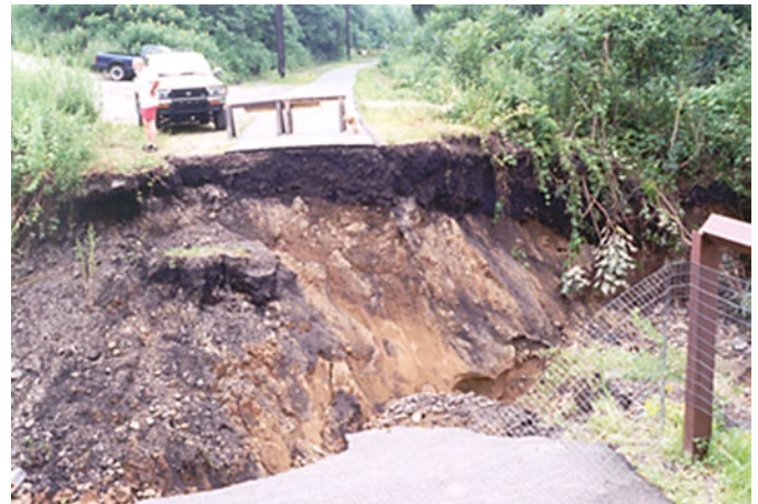
Culvert failure, Allegheny River Trail, PA.
