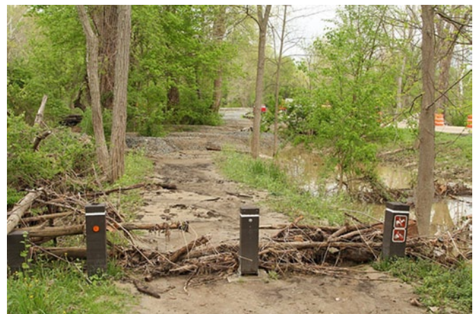
Erosion damage to stone dust trail.
