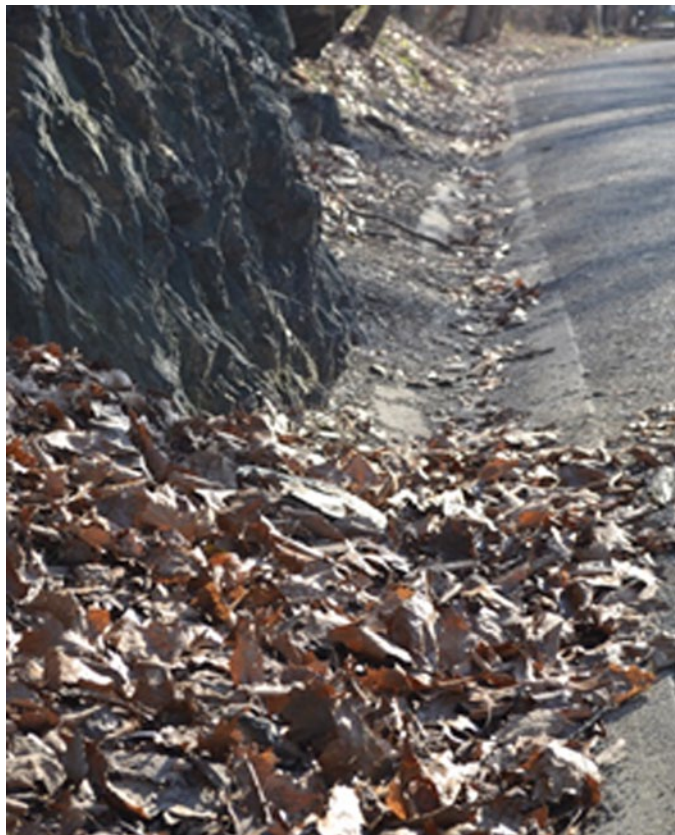
Drainage swale in need of cleaning.
