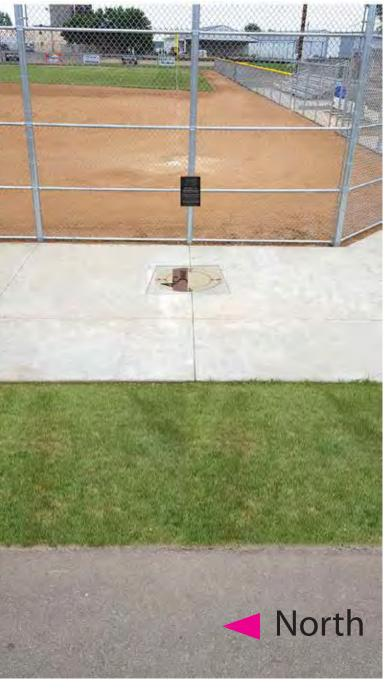
27" in Diameter disc - cast specialty concrete - flush mounted into a concrete pad constructed in the grass strip between the walking path and concrete gallery.
