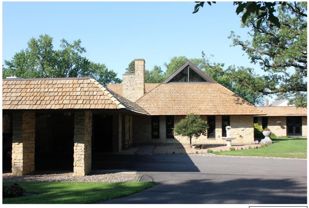
MAIN BUILDING - EAST ELEVATION INTENT IS TO MATCH EXTERIOR STONE AND WOOD SIDING & SHAKES
