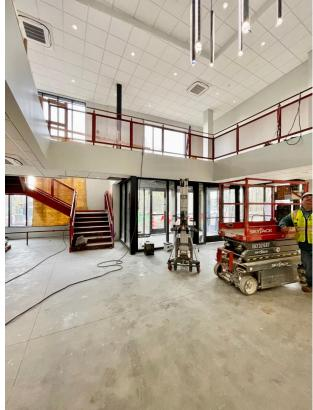
Interior spaces are starting to take shape with the installation of lighting, railings and stairs. Tile flooring and other finish work continues inside while outside crews work to prep the parking areas for paving.
