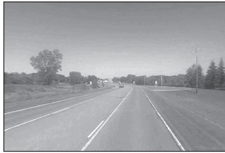
Road safety improvements that will begin in September include converting Highway 5 into a 3-lane roadway, like the one pictured above.
