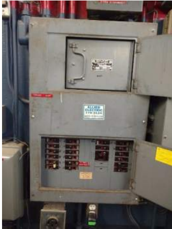
Figure FS1-O.1: Main service panel
