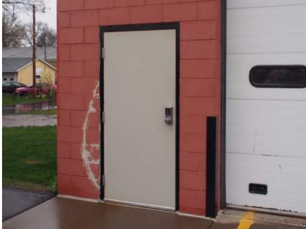
Figure FS1-C.4.b.4: Crack at man door into truck bay
