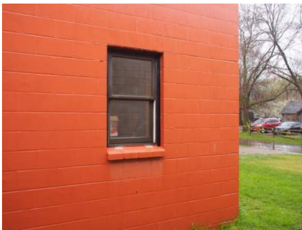
Figure FS1-C.4.b.2: Missing paint at sill
