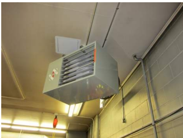
Figure FS1-M.5.a.2: Unit heater in apparatus bays
