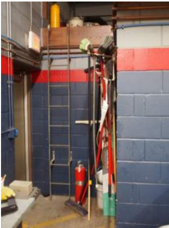
Figure FS1-E.2: Ladder not secure
