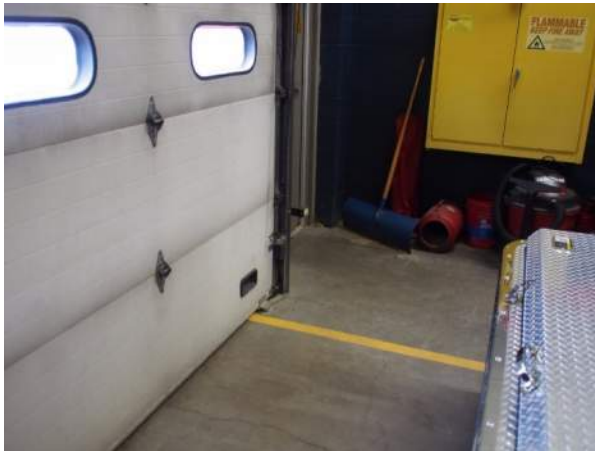
Figure FS1-H.3: Overhead doors do not meet UL325
