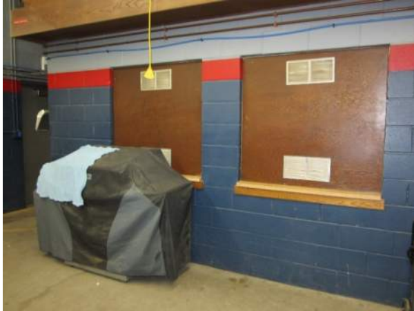
Figure FS1-M.3.a: Vents between kitchen and apparatus bay
