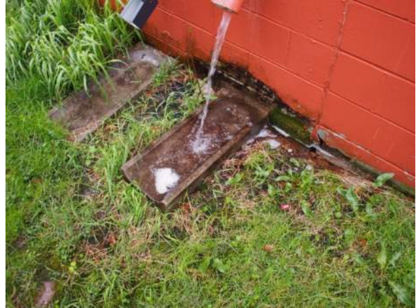
Figure FS1-C.4.b.5: Damage to block from water splashing
