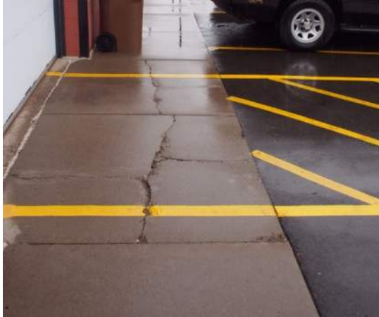
Figure FS1-B.4.b: Cracked concrete apron
