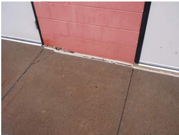
Figure FS1-C.4.d: Failing sealant at base of wall
