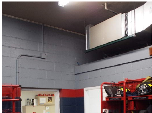
Figure FS1-M.2.a: Furnace suspended from roof structure
