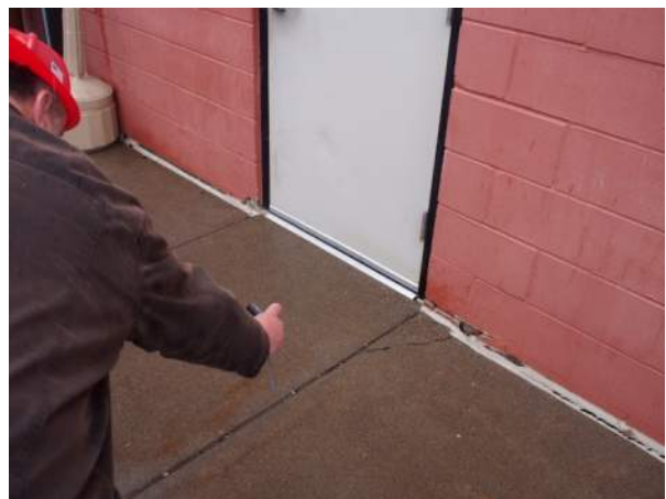
Figure FS1-C.4.b.3: Cracked block at base of wall
