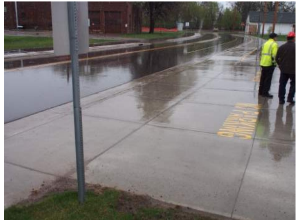
Figure FS1-G.1: No truncated dome detectible warnings
