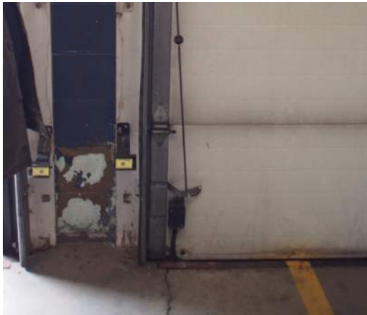
Figure FS1-D.2.a.1: Paint damaged at base of wall
