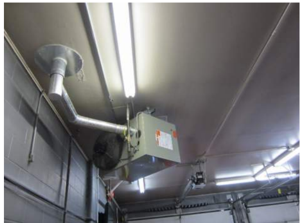
Figure FS1-M.5.a.1: Unit heater in apparatus bays
