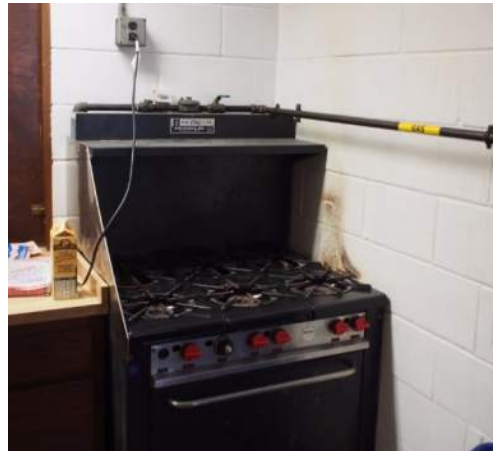
Figure FS1-D.2.a.2: Damaged paint at range
