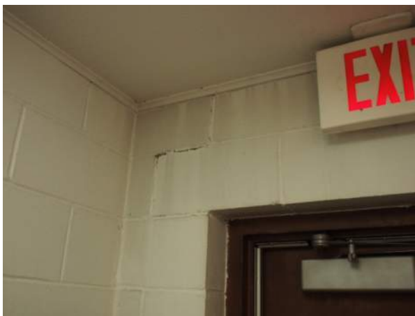
Figure FS1-D.2.a.3: Crack in masonry above side door
