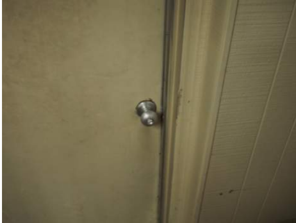
Figure FS1-G.4: Door hardware not accessible
