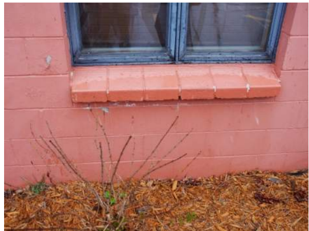
Figure FS1-C.4.b.1: Peeling paint by windows
