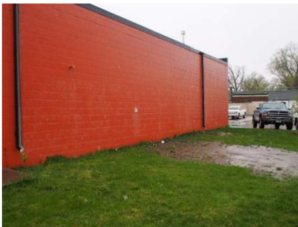
Figure FS1-B.2.b: Missing splashblock
