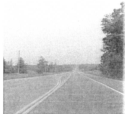
Inwood Ave. Near 15th St., Looking North
