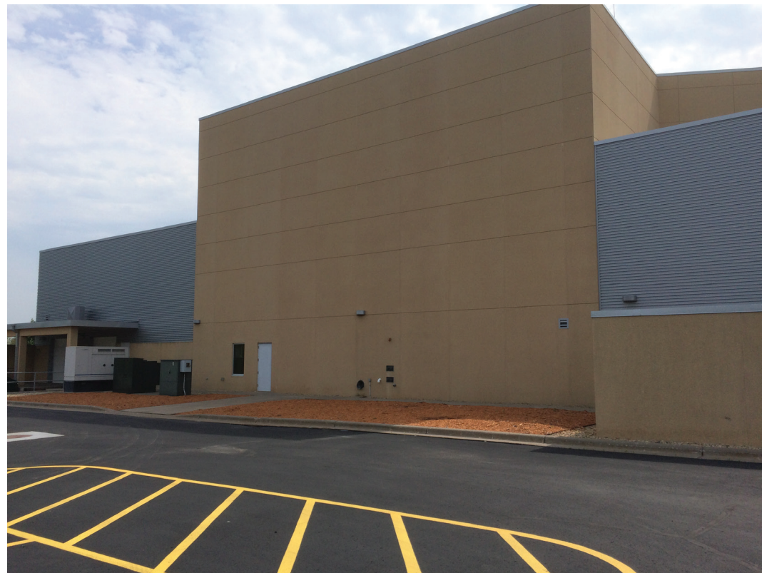
PHOTO REFERENCE AT THE NORTH END OF THE EXISTING BUILDING LOOKING SOUTH
