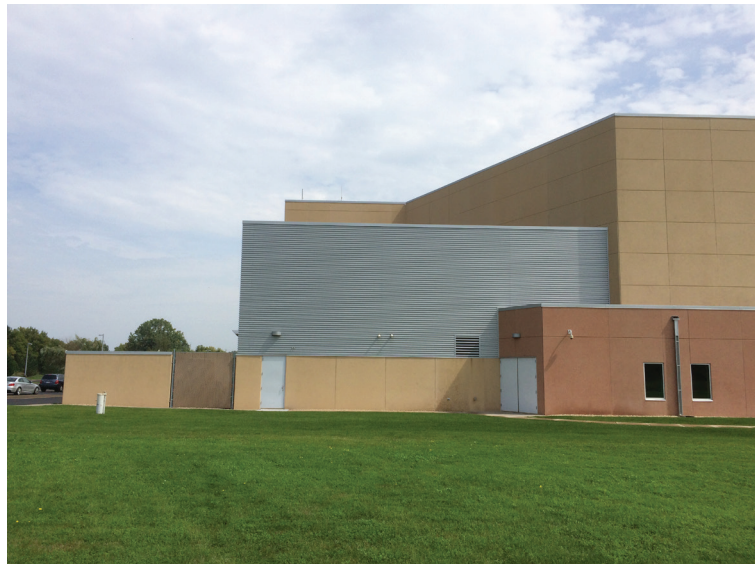
PHOTO REFERENCE AT THE NORTH END OF THE EXISTING BUILDING LOOKING EAST
