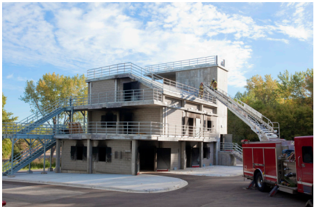
ABLE Burn Building
